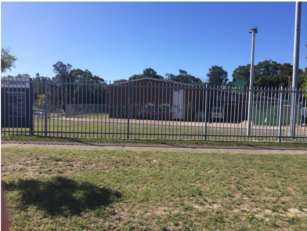
Photo 2 | The Site looking north at exchange building
